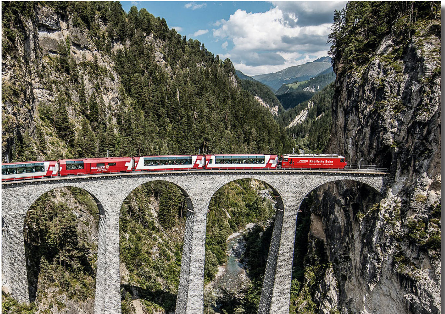
EXCELLENCE CLASS, Rhaetian železnice Landwasser Viaduct, Švýcarsko EXCELLENCE CLASS, Rhaetian Railways Landwasser Viaduct, Switzerland
