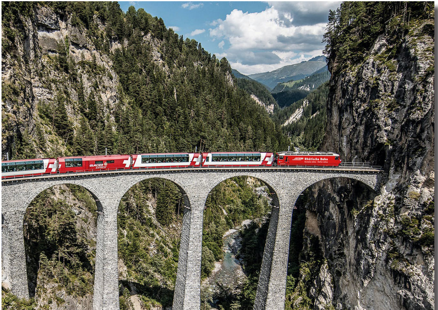
EXCELÊNCIA, Rhaetian Railways Landwasser Viaduct, Switzerland EXCELLENCE CLASS, Rhaetian Railways Landwasser Viaduct, Switzerland
