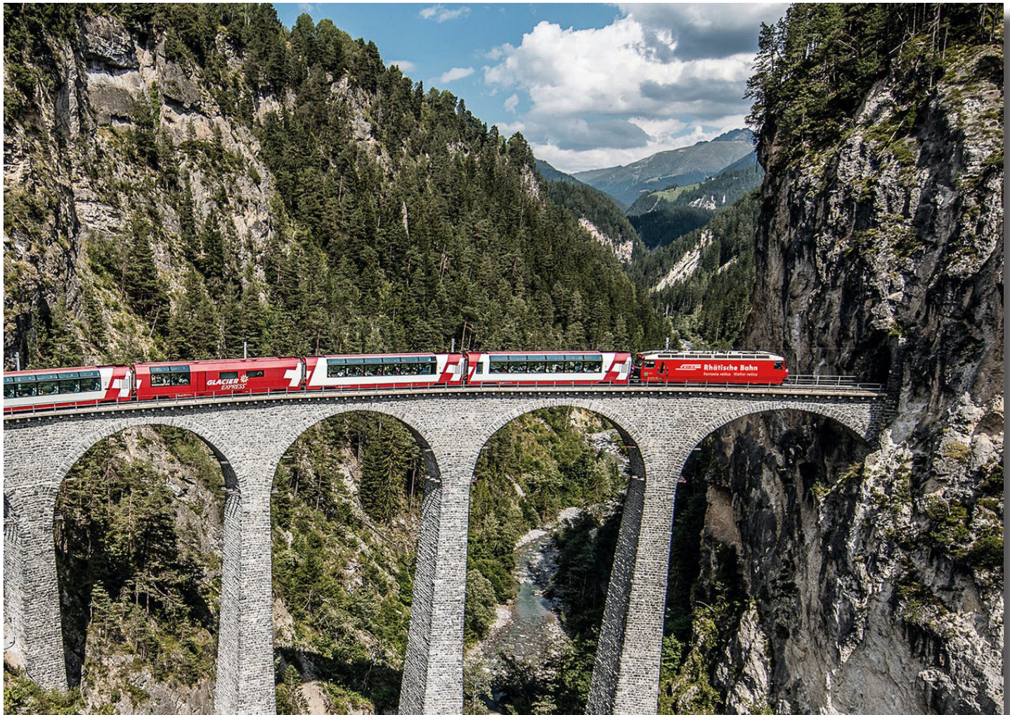
卓越级 瑞士雷泰铁路朗瓦瑟高架桥 EXCELLENCE CLASS, Rhaetian Railways Landwasser Viaduct, Switzerland
