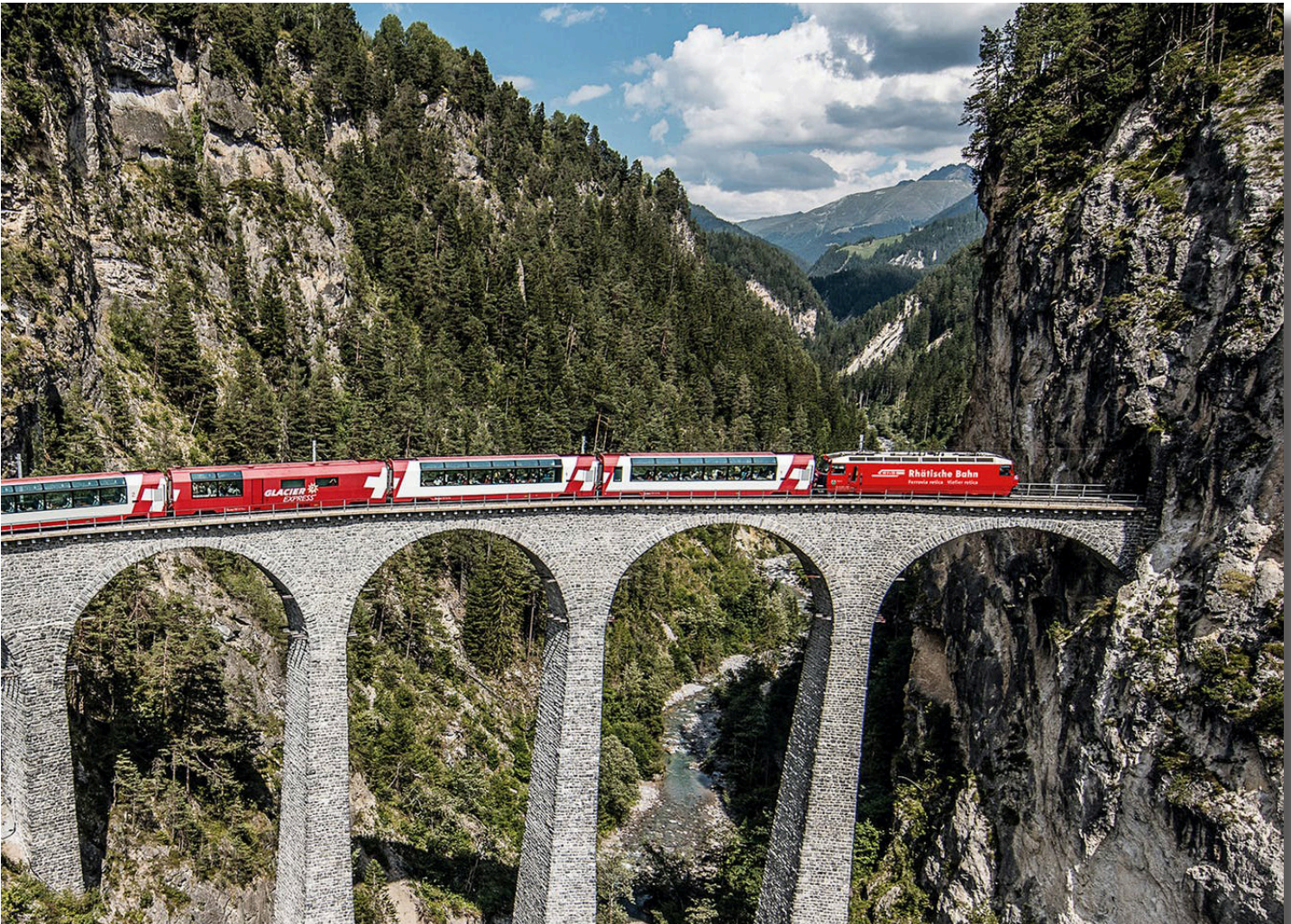
Excellence Class, Rhaetian Railways Landwasser Viaduct, Switzerland
