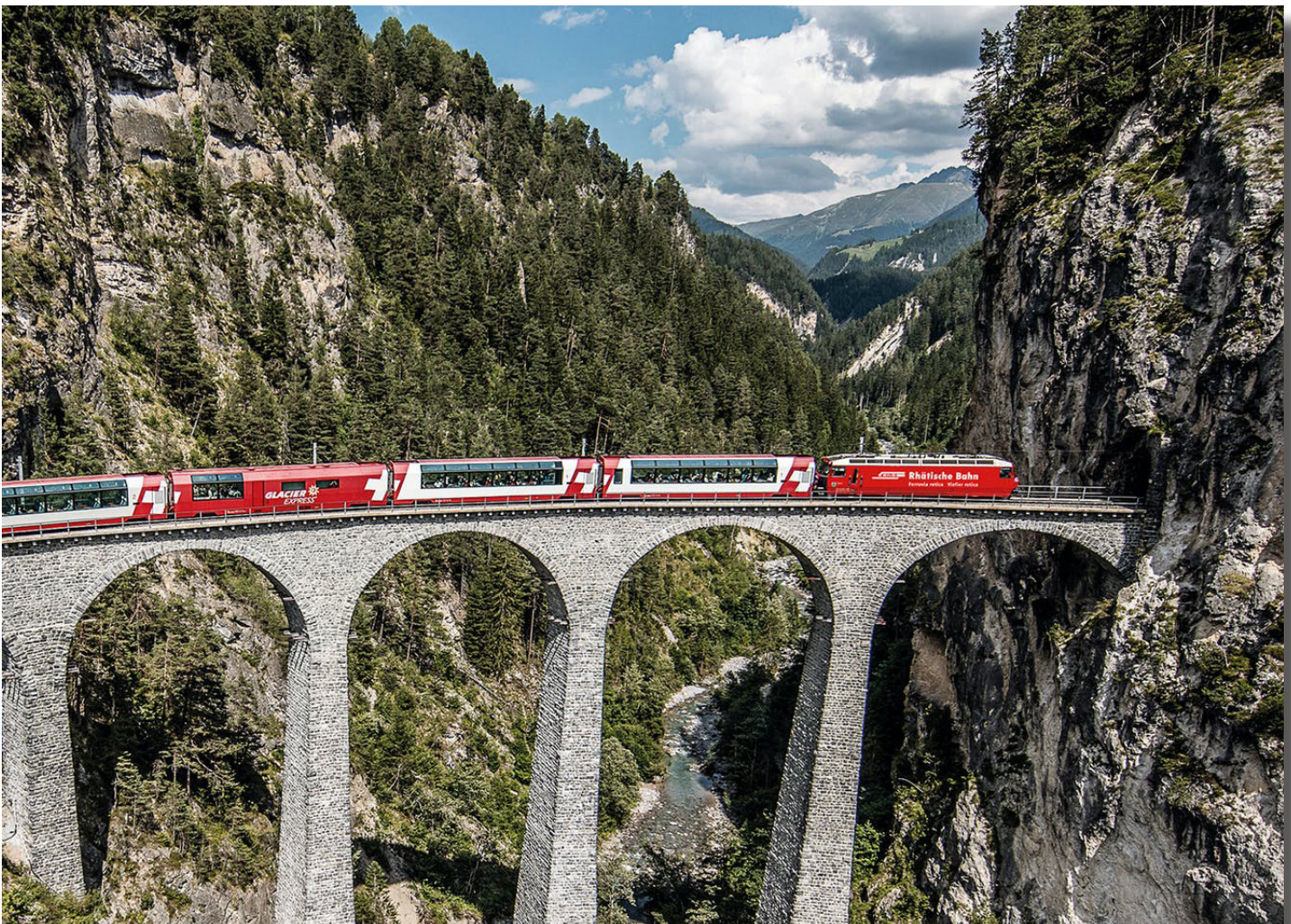
Excellence Class, Rhaetian Railways Landwasser Viaduct, Switzerland
