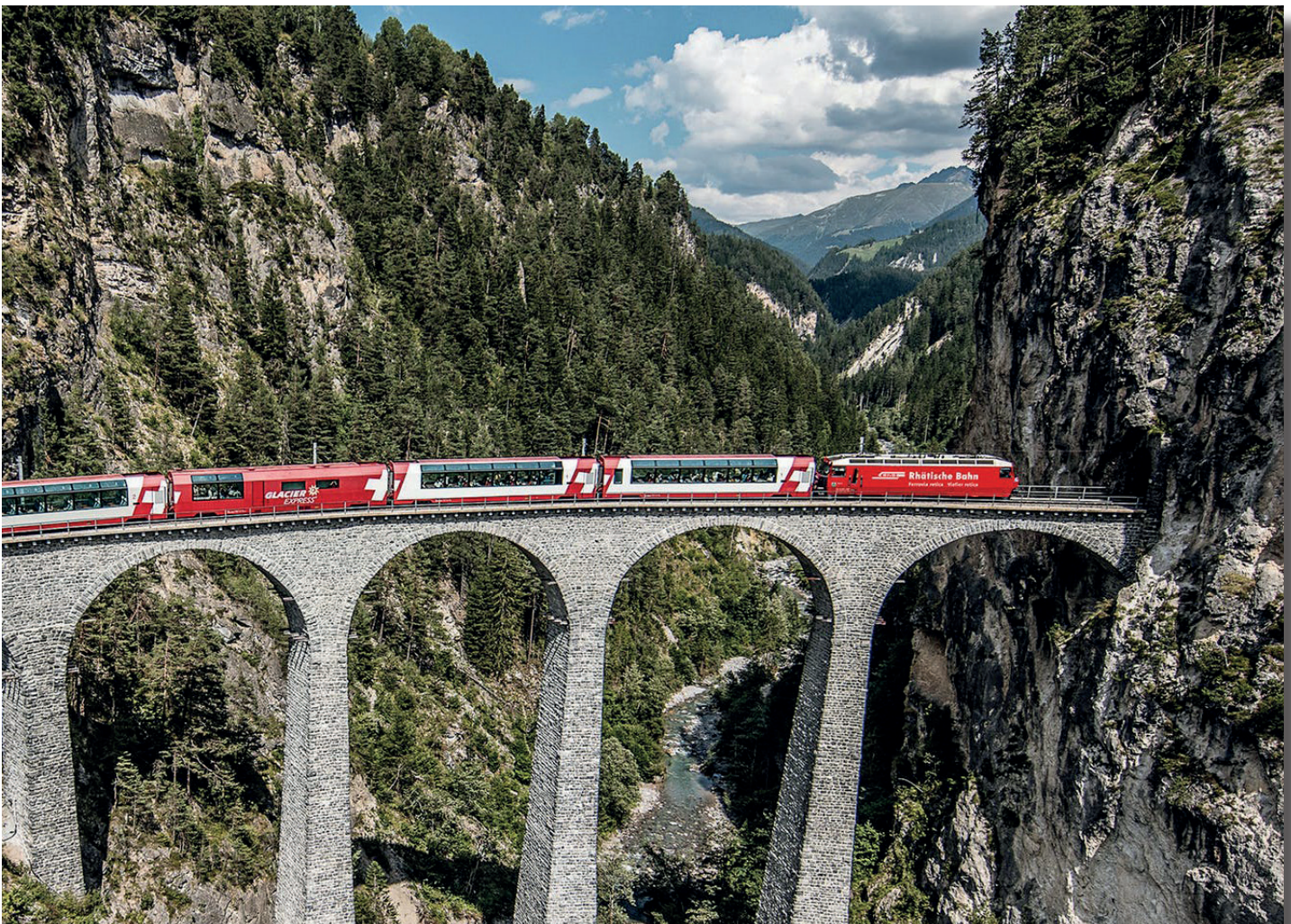
Excellence Class, Rhaetian Railways Landwasser Viaduct, Switzerland
