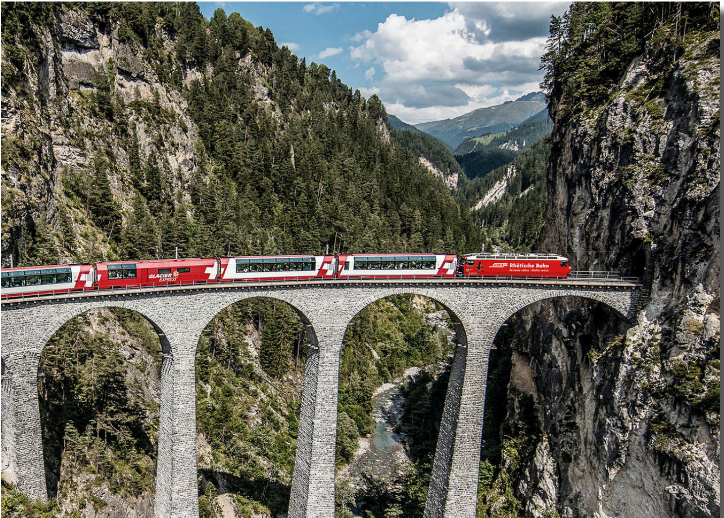
Excellence Class, Rhaetian Railways Landwasser Viaduct, Switzerland
