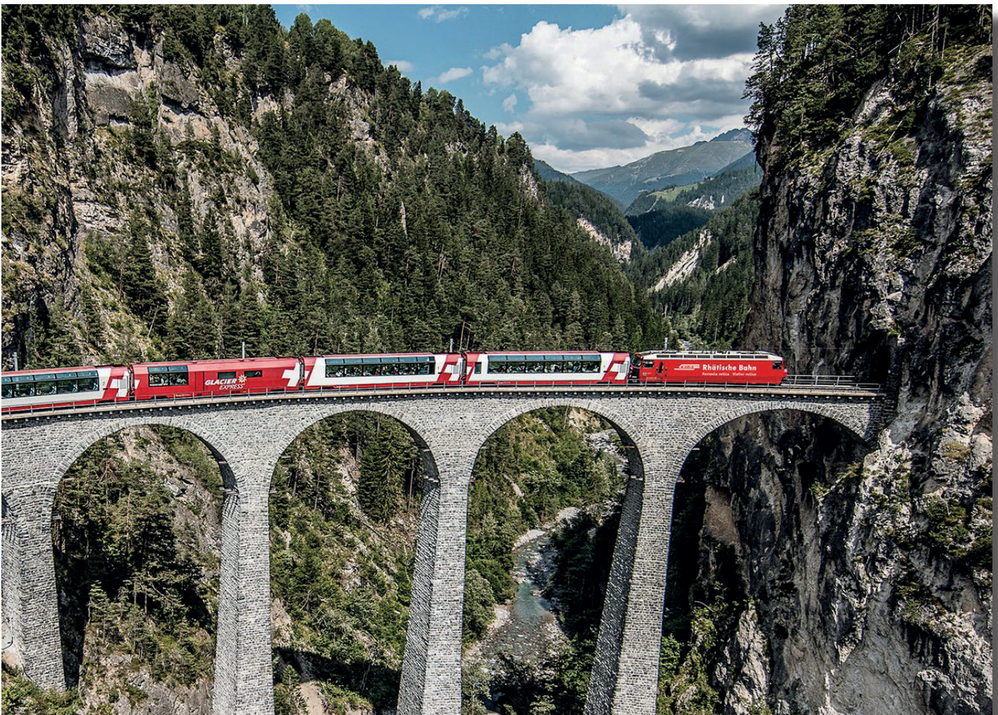
Excellence Class, Rhaetian Railways Landwasser Viaduct, Switzerland
