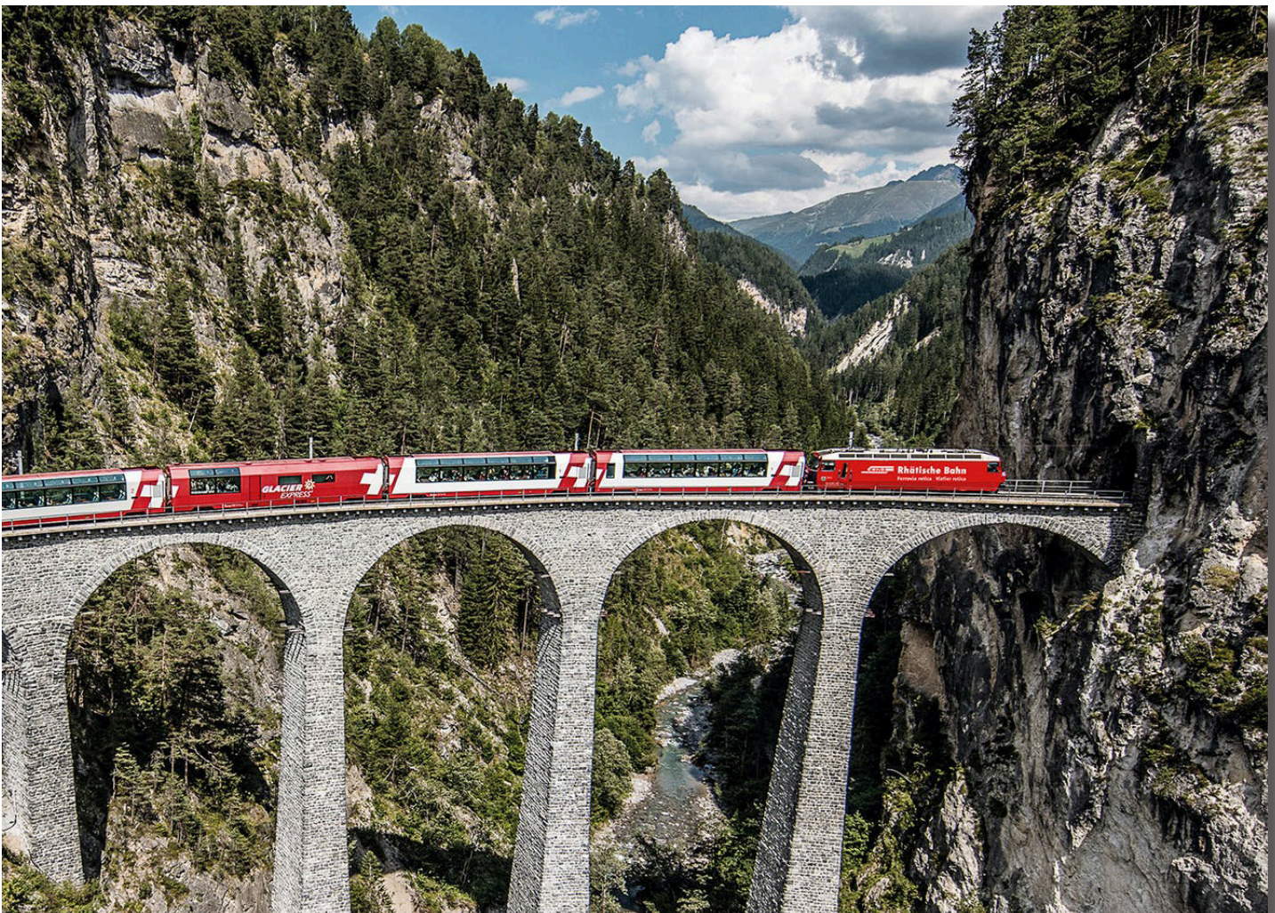
Excellence Class, Rhaetian Railways Landwasser Viaduct, Switzerland
