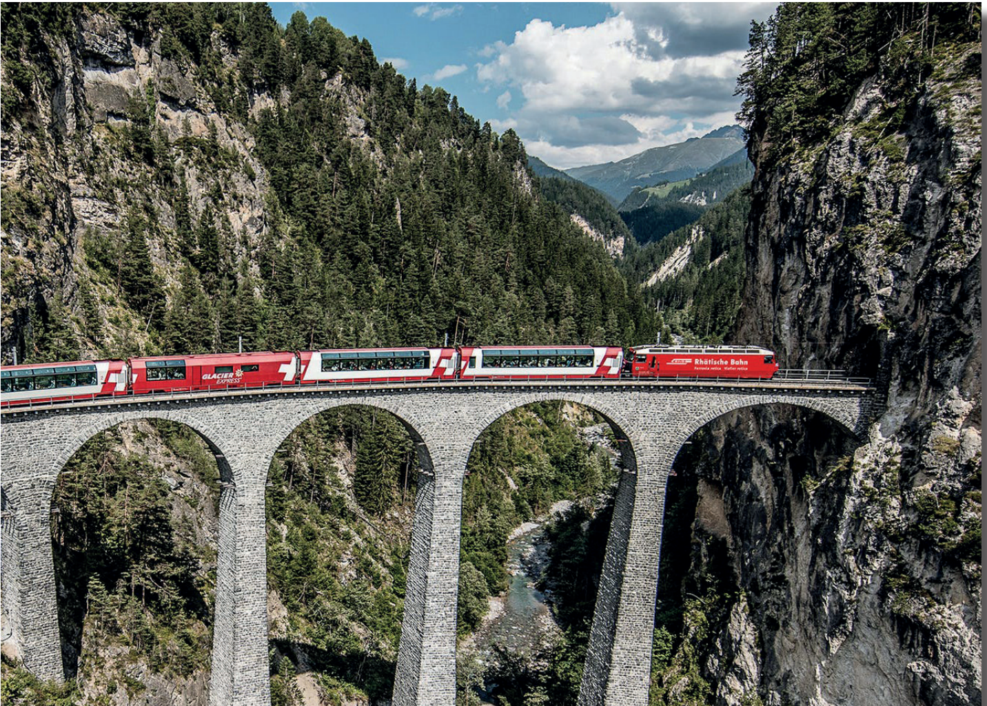
Excellence Class, Rhaetian Railways Landwasser Viaduct, Switzerland
