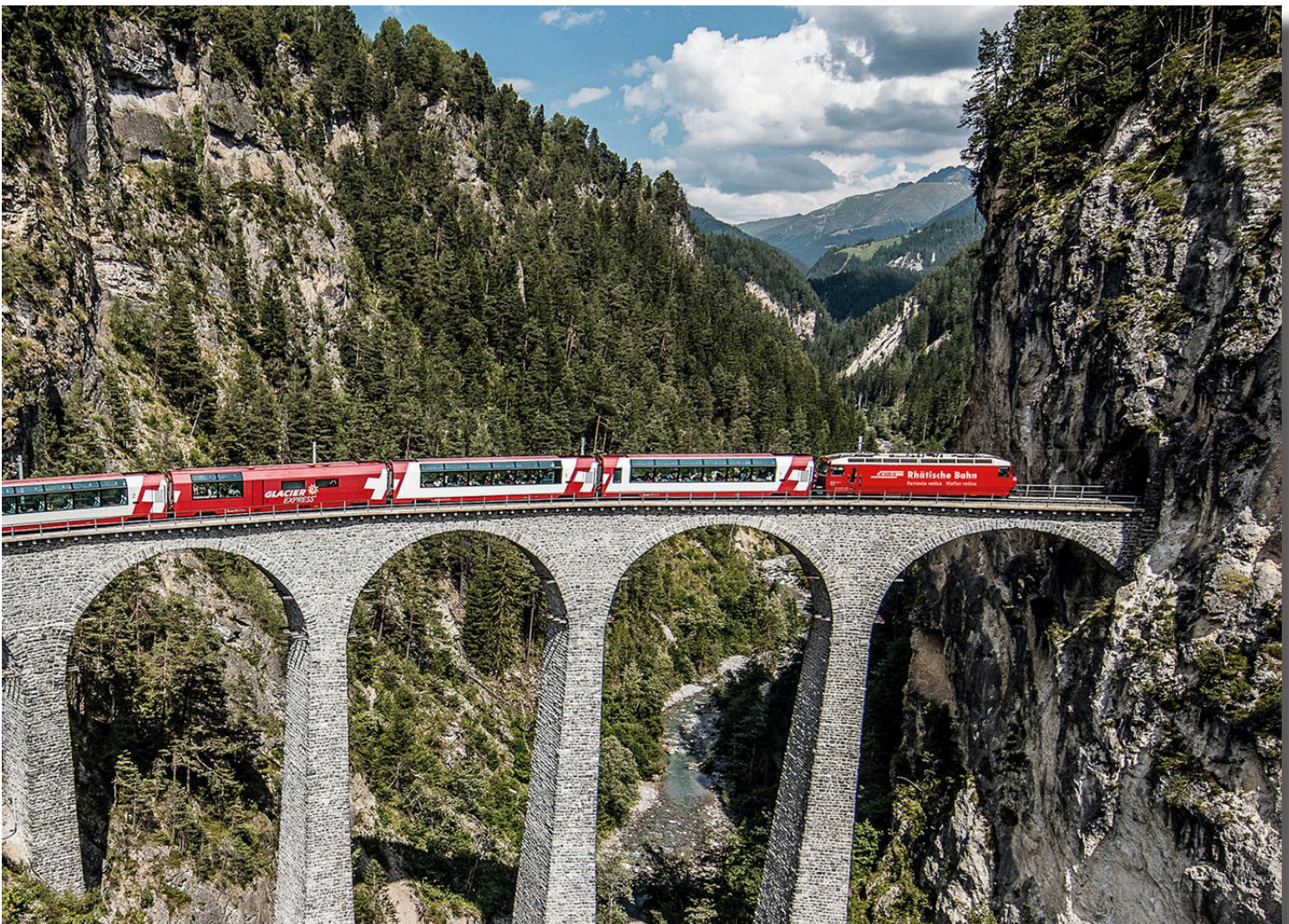
Excellence Class, Rhaetian Railways Landwasser Viaduct, Switzerland
