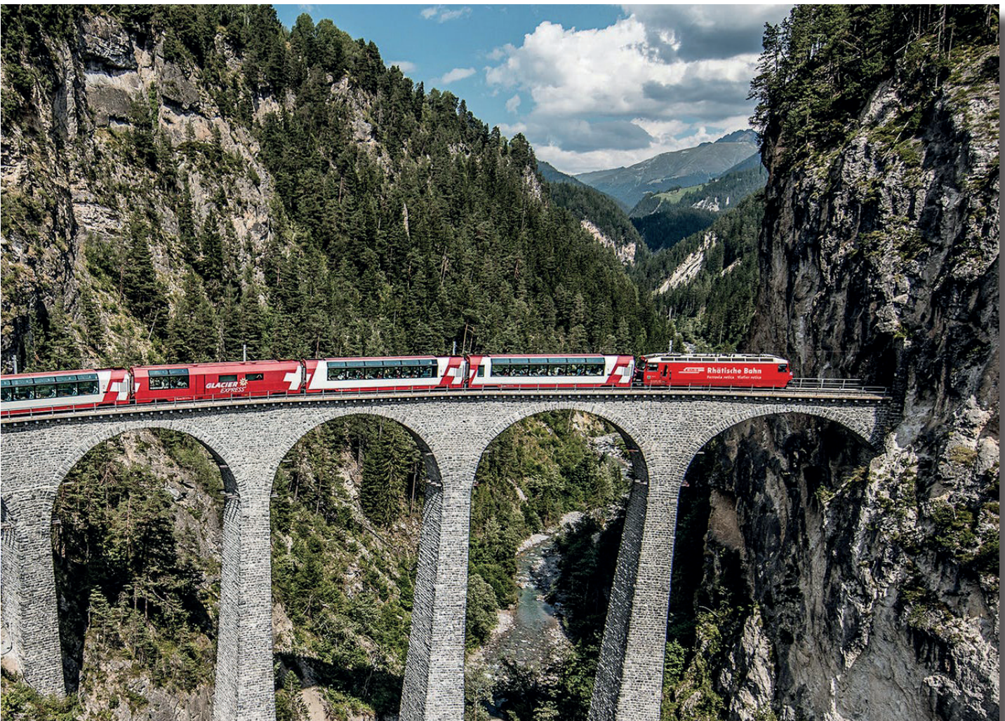
Excellence Class, Rhaetian Railways Landwasser Viaduct, Switzerland
