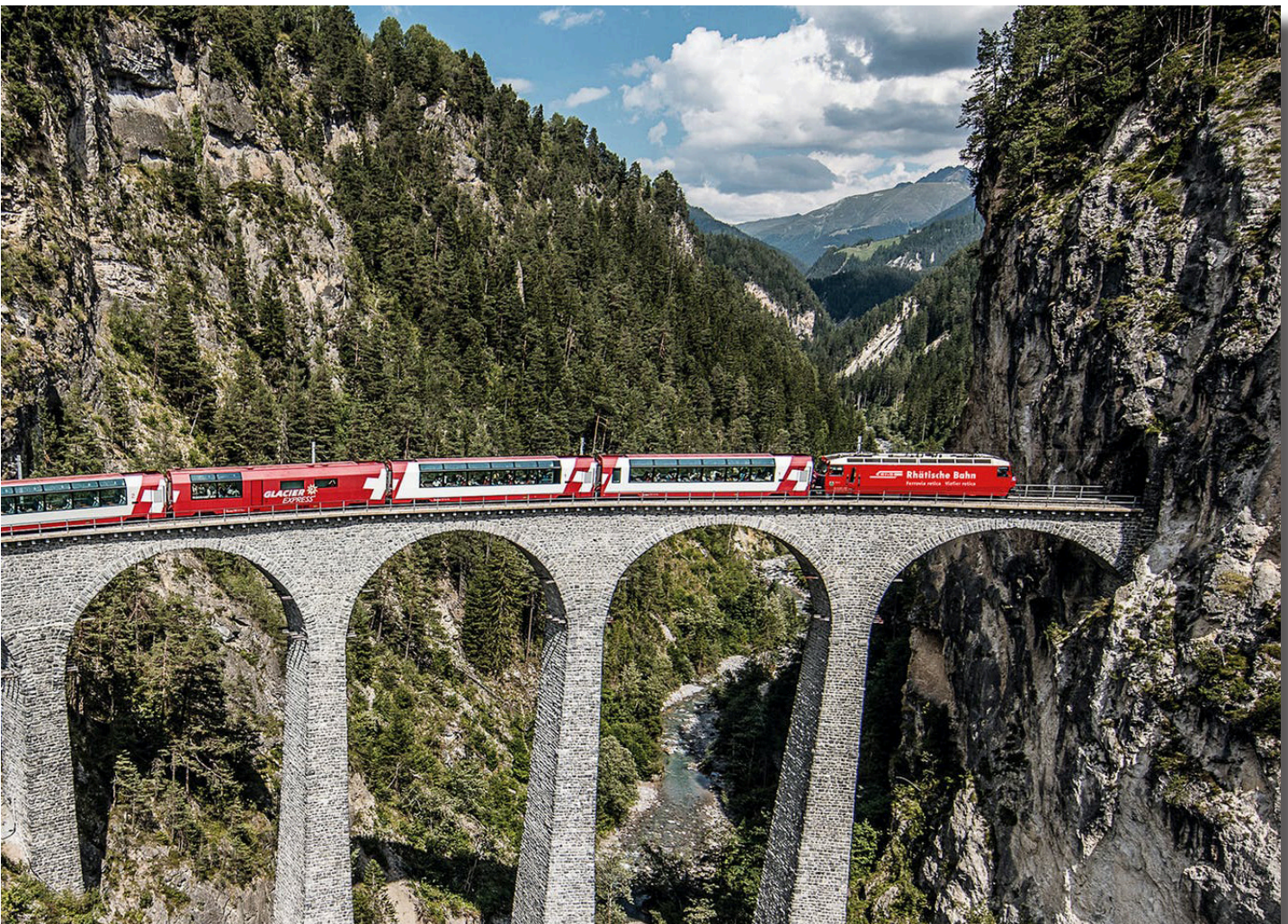
Excellence Class, Rhaetian Railways Landwasser Viaduct, Switzerland
